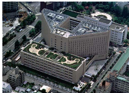
St. Luke's International Hospital
