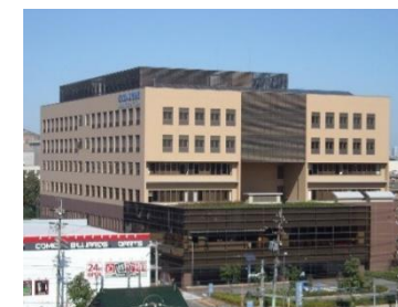
Nagoya District Court
