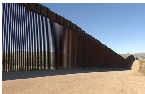
The border wall under construction between the United States and Mexico
